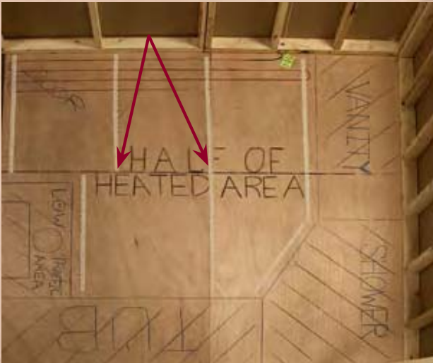
FIGURE 4a 30" distance between adjacent rows of strapping
