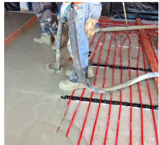
Its special formula resists breakdown up to 150°F (66°C). And because it's poured only 1-1/4" to 1-1/2" (32 mm to 35 mm) thick, the heating system is more responsive and more comfortable.
