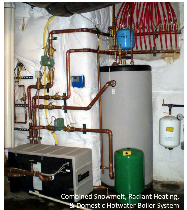
Dedicated Lochinvar High Efficiency Snowmelt Boiler
