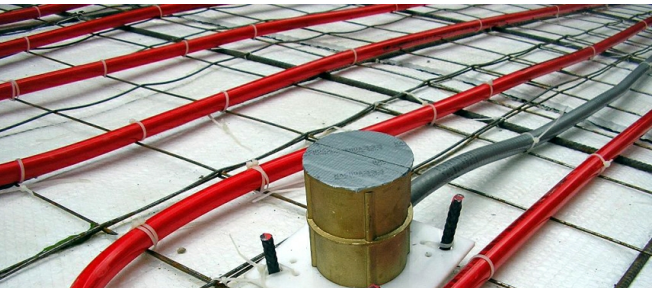
Snow Detection Slab Sensor in a hydronic snowmelt system
