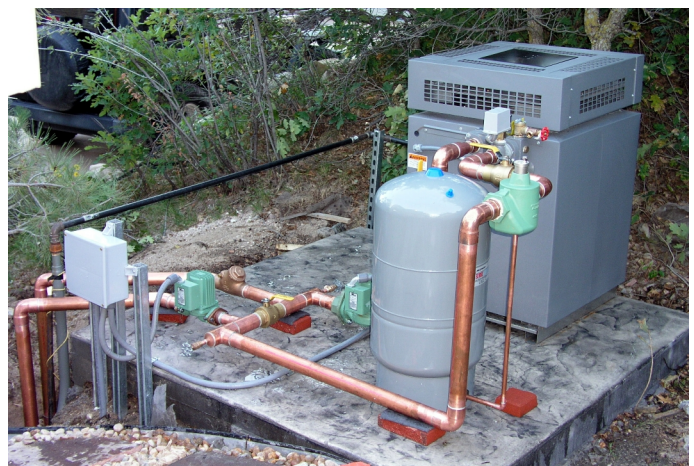
Pictured above is a snowmelt boiler system designed to be placed outdoors. Weather-proofing must be considered in the design application of this system. This is a great option for when indoor space is not available.
