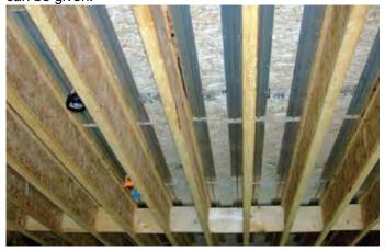
Once the surface preparation of the subfloor area is made the installer can screw or staple **Radiant Side Trak**<sup>TM</sup> to the subfloor. **Radiant Side Trak**<sup>TM</sup> comes with 10 prepunched openings per panel if screws are to be used. Staple and screws lengths should not exceed ¾". If a pneumatic air gun is available, you could use ¾" -16 gauge construction staples. Staples or screws should have 10 per panel, 5 per side.
