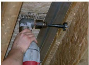
For engineered floor systems (TJI), you can utilize knock out holes provided in the same fashion. Truss flooring systems will present less of a problem. The only caution in Truss flooring is the sharpness of the fastener as they have a tendency to be sharp and can cause a breach in the tubing wall. It can also peel the EVOH barrier off Pex.
