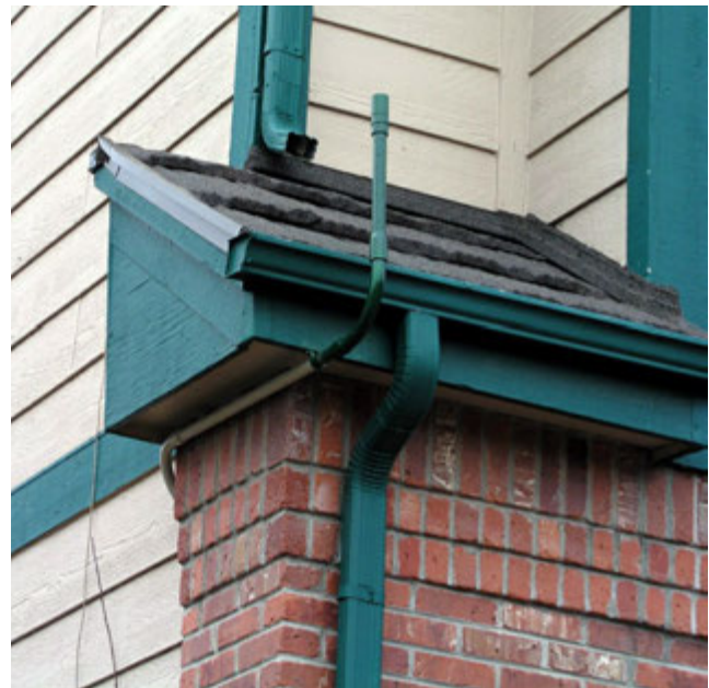
Pictured above is an aerial-mounted remote sensor for an automatic snowmelt control system. When snow accumulates on the sensor, it activates the system. A pavement-mounted version is also available (shown on page 15).
