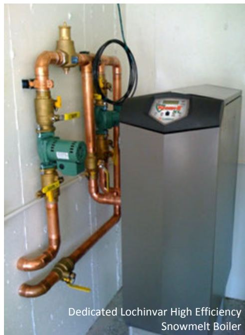
Dedicated HTP High Efficiency Snowmelt Boiler
