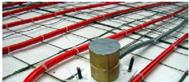
Snow Detection Slab Sensor in a hydronic snowmelt system
