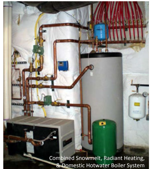
Dedicated Lochinvar High Efficiency Snowmelt Boiler
